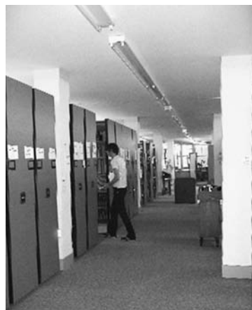
Completed compact shelving
